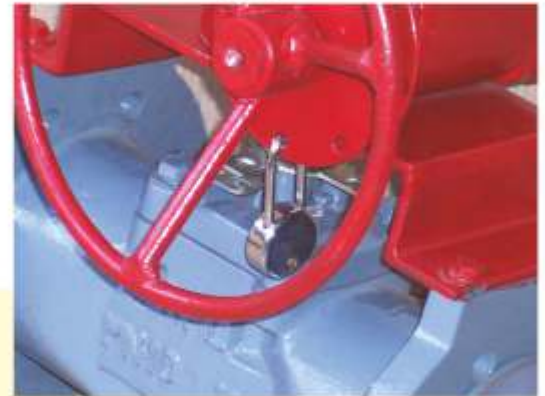
Gear with locking provision
