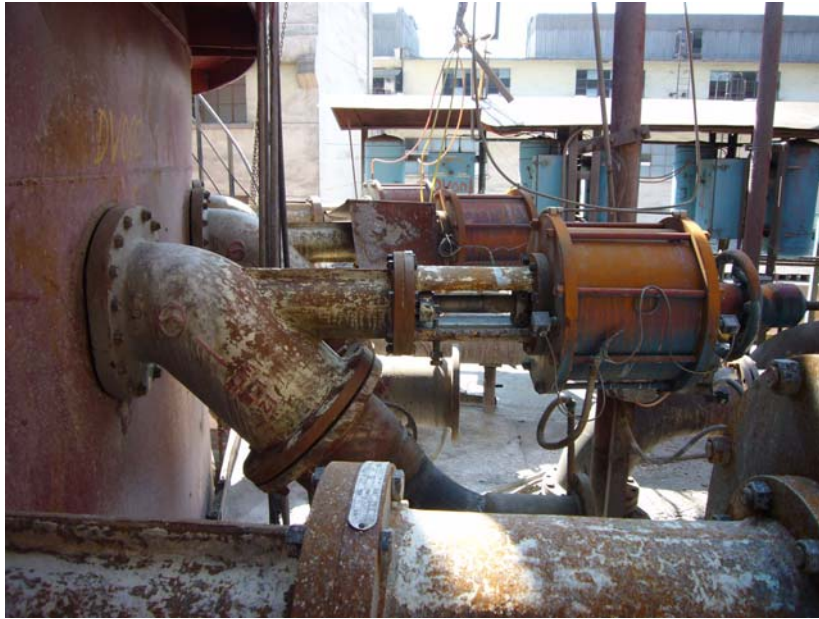
Pneumatic dumping valve used in alumina
