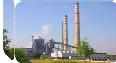
Thermal power plants
