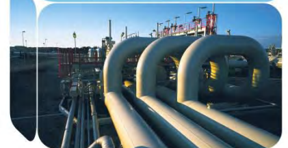
West-east gas pipeline
