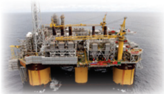
Planta Off-Shore (Noruega) Off-Shore plant (Norway)
