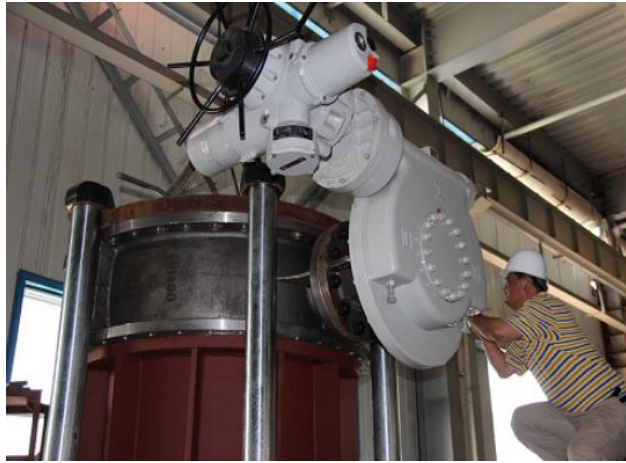
Pressure testing by customer CNOOC
