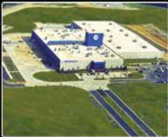
PAGELAND, SC Bronze Foundry and Manufacturing Plant
